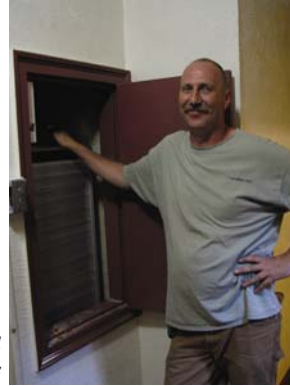
Skip is happy that the dumbwaiter installation is complete!
